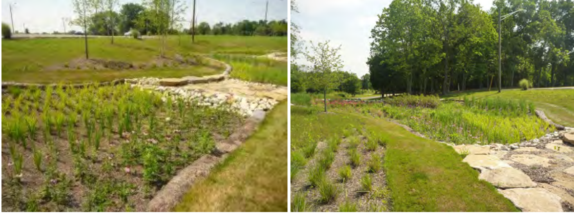
Figure 124. Bioretention Basins (stormwater.wef.org)
