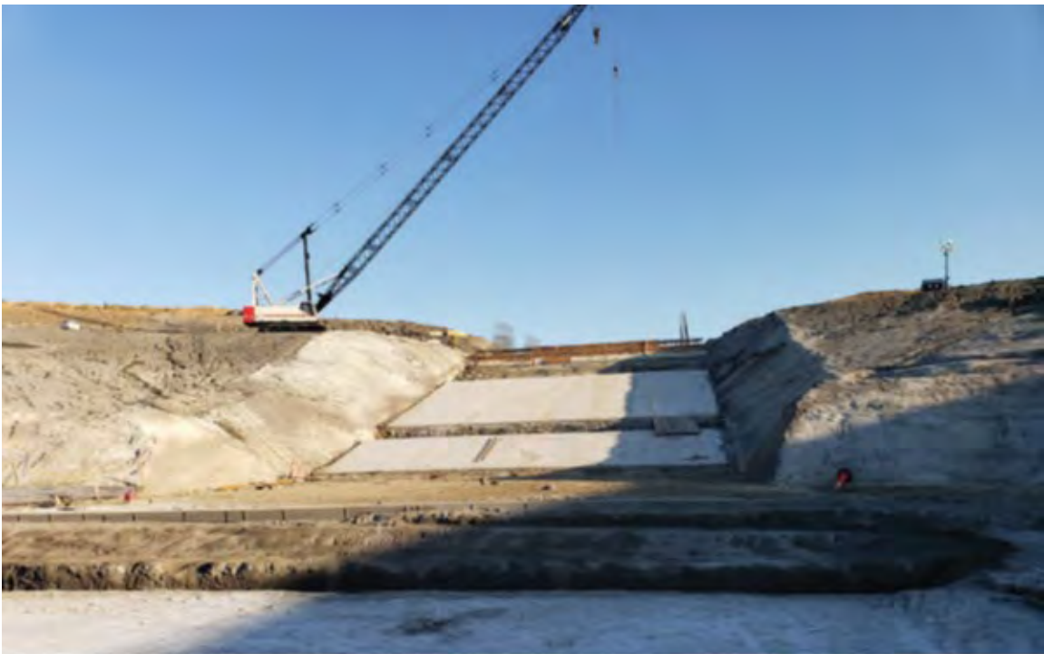
Figure 1-1. Constructing the Dam Spillway, June 2019
