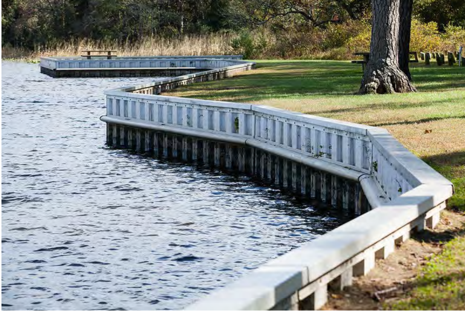
Figure 3. Shoreline Bulkhead Examples (chesapeakebay.net)
