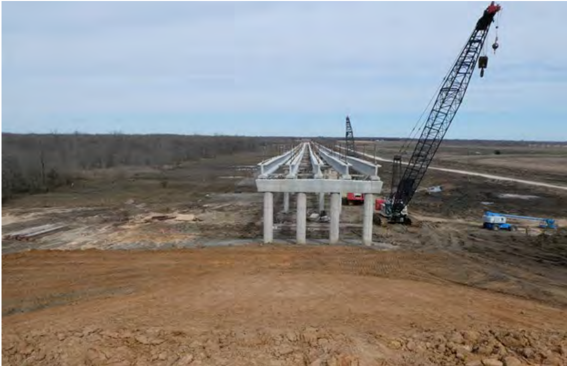
Figure 1-2. Farm-to-Market Road 897 Crossing Future Reservoir (Looking North)
